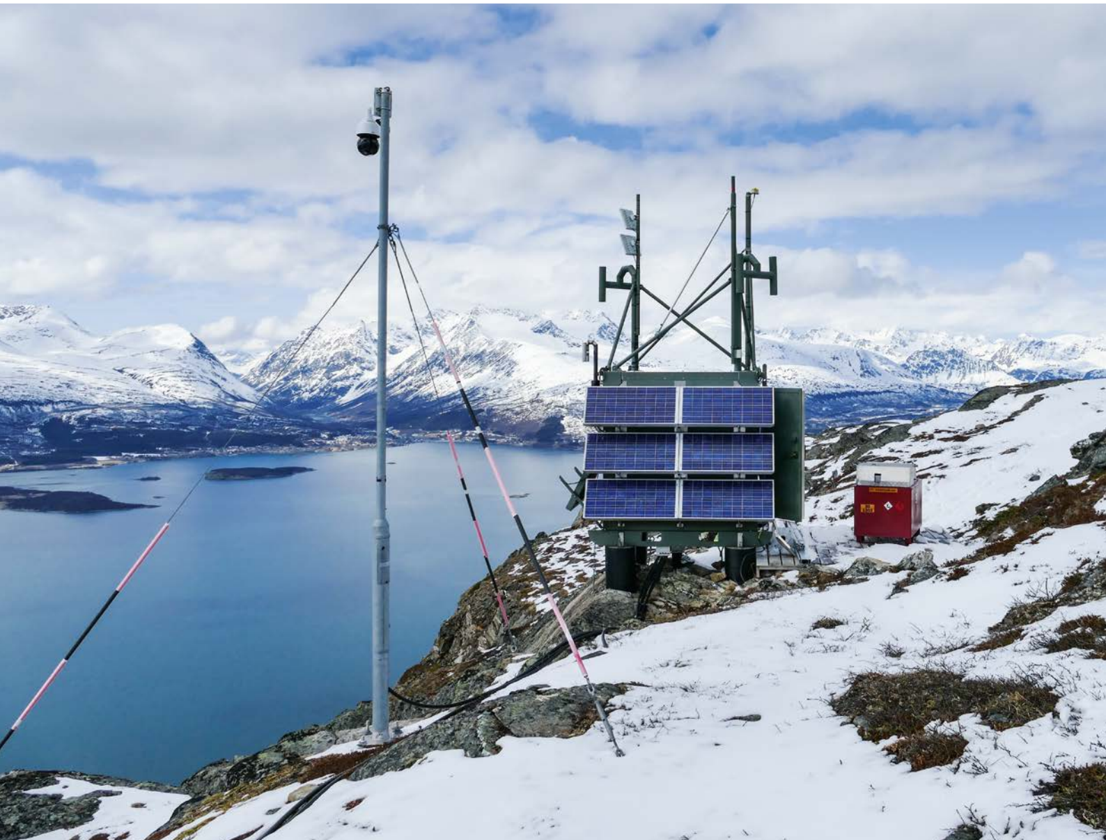
Off-grid is a success: Fuel cells have proven themselves in off-grid applications, such as this landslide monitoring station. © SFC Energy
