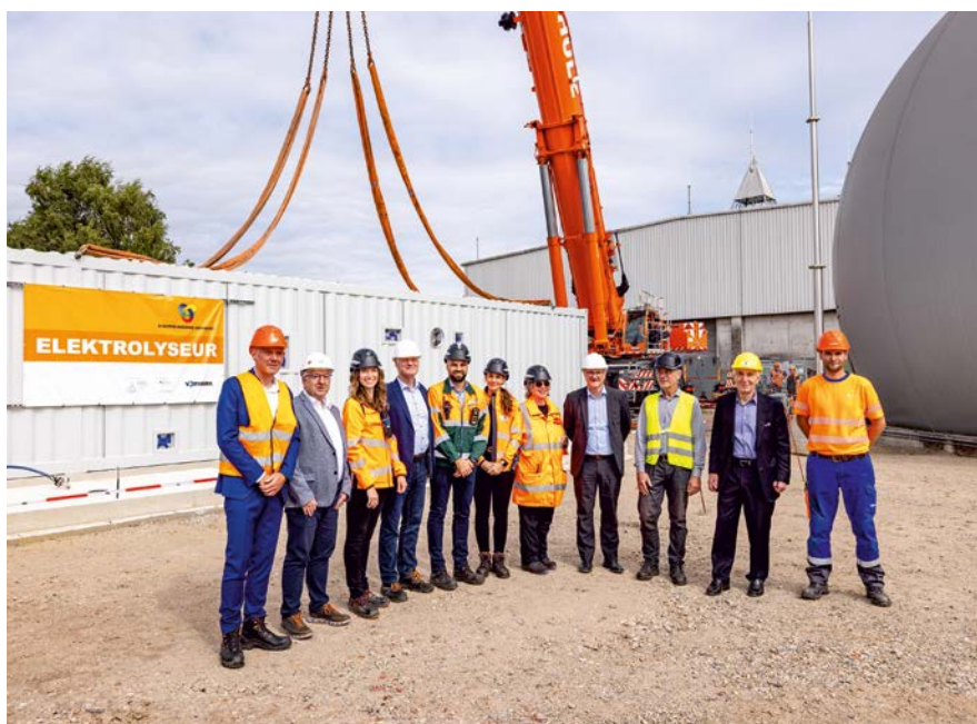
The Managing Director of Stadtreinigung Hamburg, Prof. Rüdiger Siechau (second from right), with the project team in front of the new electrolysis plant.
