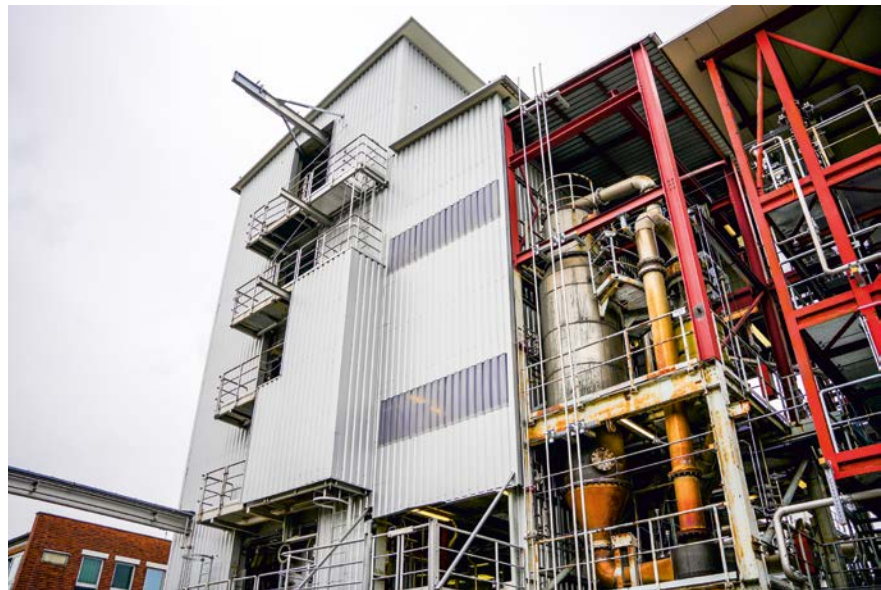
The Circored pilot plant in Frankfurt, Germany is intended to produce sample material on a ton scale for potential customers © Metso
