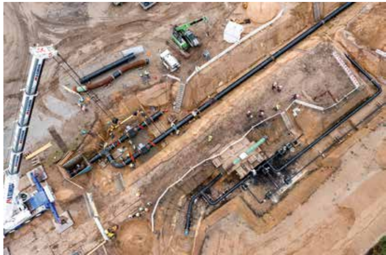
Fig. 1: Installation of the pig launching station at Ontras' Bad Lauchstädt energy park in November 2023. [Source: Ontras]
