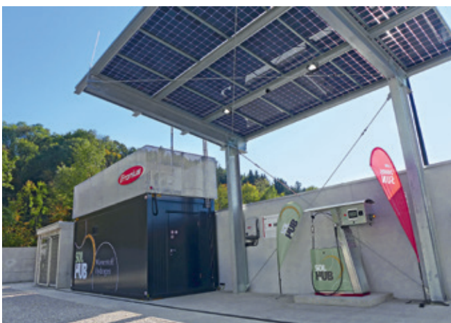
Fig. 1: The SOLH 2 UB container houses a fuel cell to generate electricity, an electrolyzer to produce hydrogen and a storage device to make use of waste heat. [Source: Joachim Berner]
