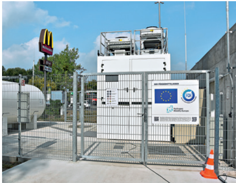
Fig. 3: The container houses an ionic compressor by Linde, as well as a stationary hydrogen tank (left).
